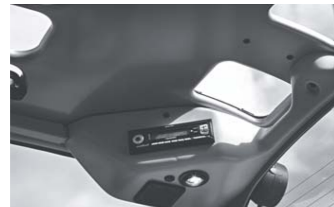
Viewing window also to the top rear in order to prevent roller shutter damage
